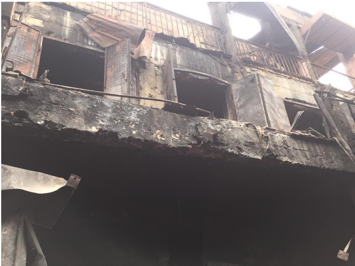
Figure 1.1 Overview of the Structure
